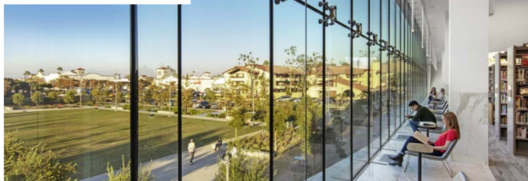
USA Donald Dungan Library, California / Data & Flooring ConCore 1250, 1500 & 2500
